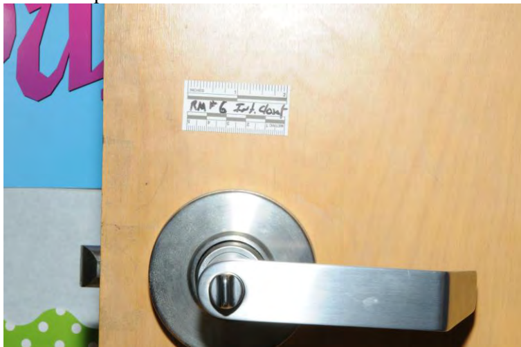
134 Example classroom closet door lock – interior
