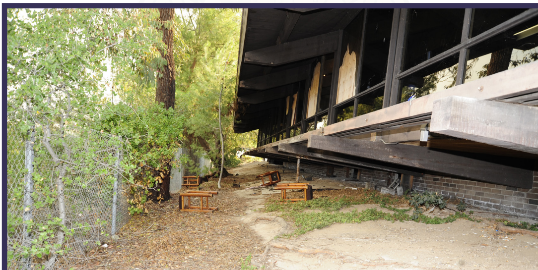
Photo 5: Photo depicts the north side of the bar. This is the location where numerous patrons/employees jumped out the windows. Opposite (or north of) the chain link fence is the on-ramp to the U.S. 101 Freeway (southbound).
