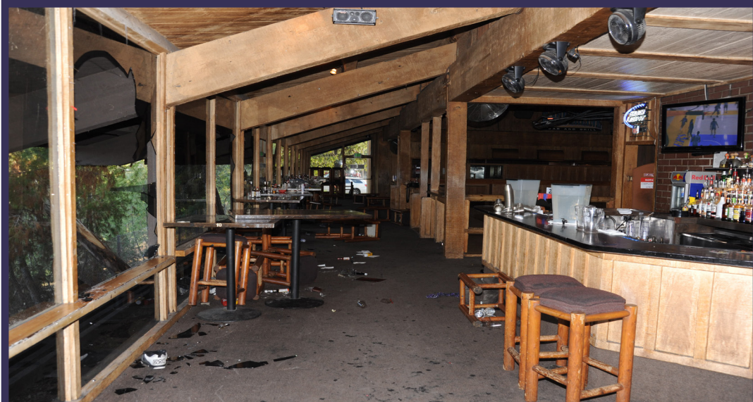
Photo 4: Photo of the glass windows along the north side of the Borderline Bar and Grill.
