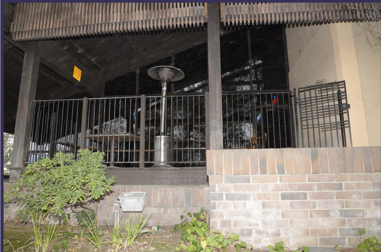
Photo 10: Photo depicts the west side of Borderline Bar and Grill (smokers' patio) and the pedestrian door several officers entered during the Secondary Entry.
